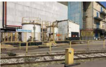
Erdemir Cold Rolling Mill Chromium Reduction Facility Capacity Increase
