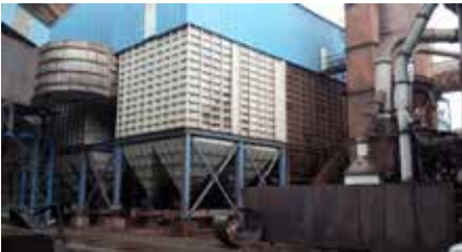
Erdemir Modernization of Sinter Plant Raw Material Dust Collection System
