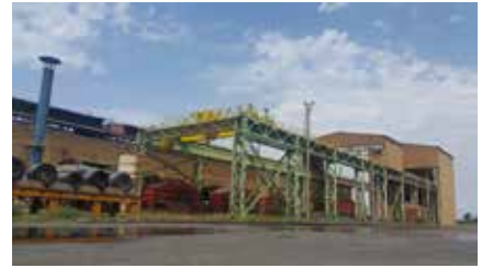
İsdemir Extension of the Scale Crushing Plant
