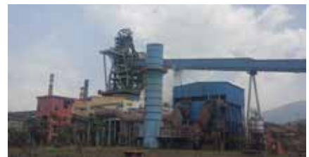
İsdemir Blast Furnace Front Dust Collection Pneumatic Pipeline
