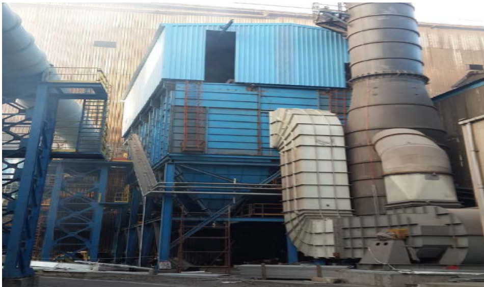
Installation of a New Dedusting System at the Desulfurization Plant
