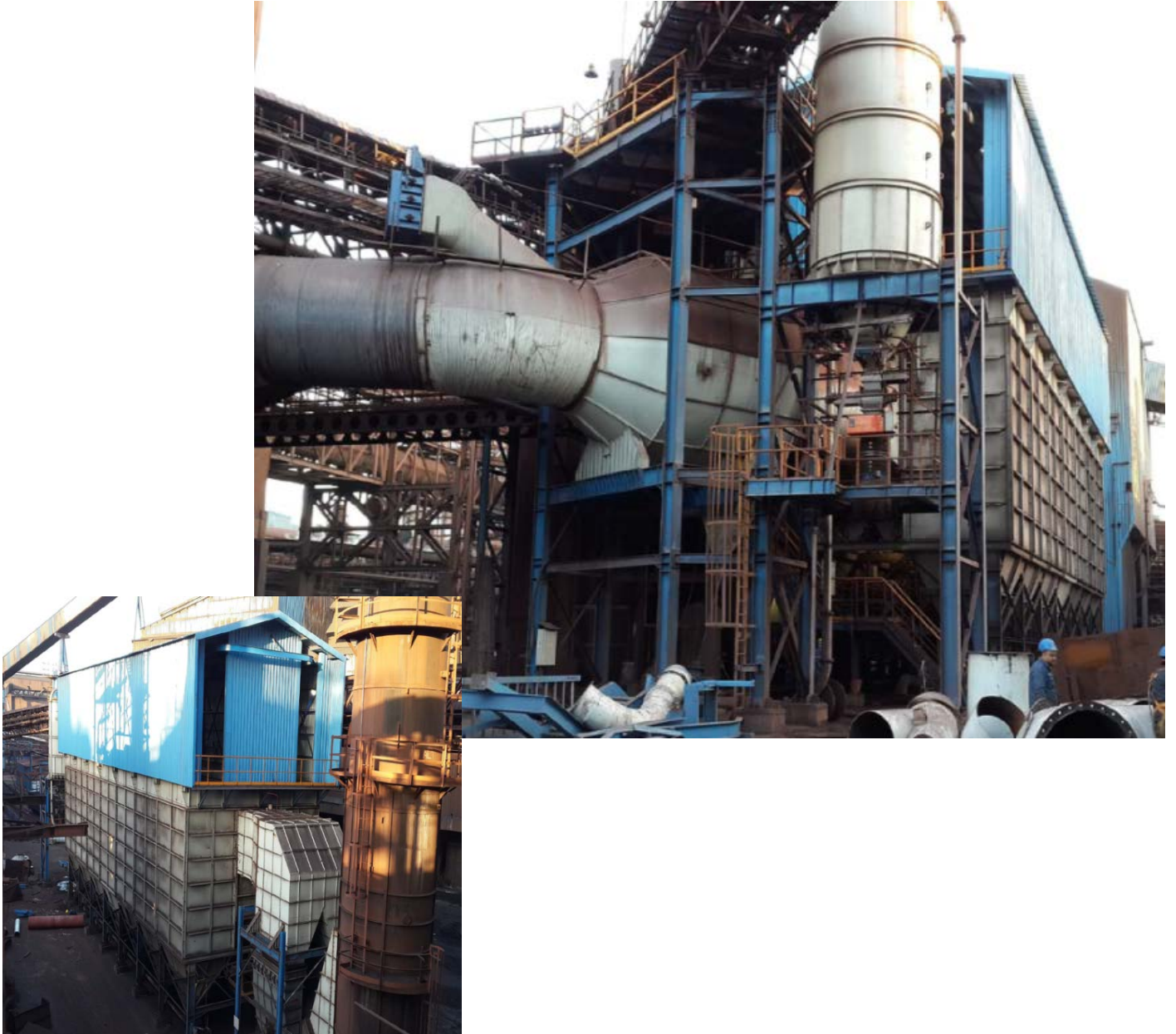
Improvement of the No. 1 Blast Furnace Foundry's Dedusting System
